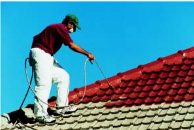
Application of Decragard Roof Coating System
