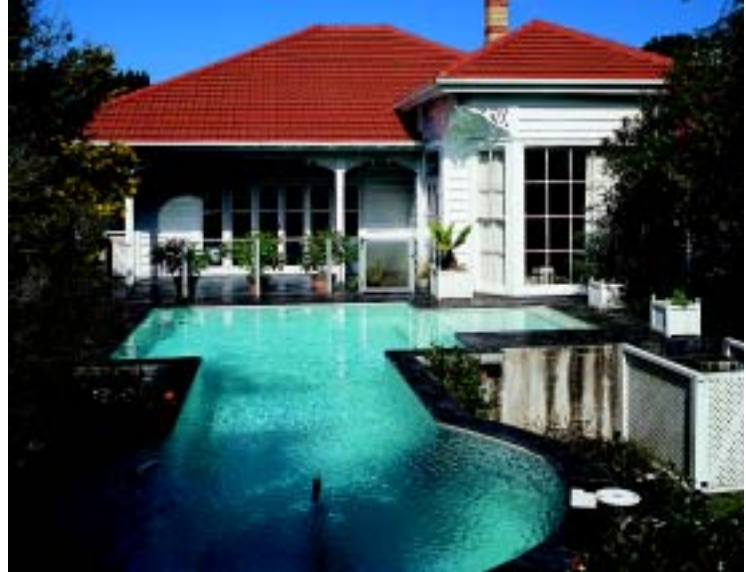
Decragard Roof Coating Systems: Before (inset) and After.
