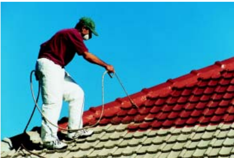
Application of Decragard Roof Coating System
